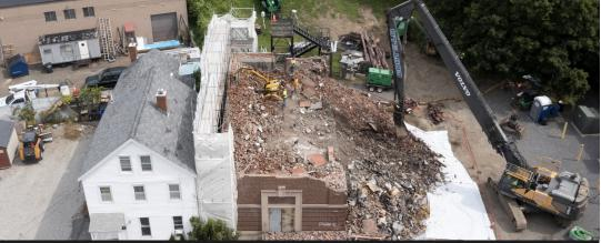
Volvo 480 High Reach Excavator assisting Brokk Robotic Excavator
