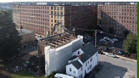
Demolition of the substation showing the western wall protection
